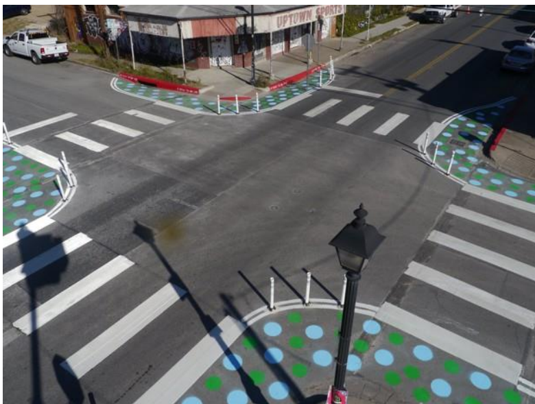
Figure 12 - The pedestrian emphasis corridors are ideal locations to implement near-term and lower cost enhancements to calm traffic, such as these temporary curb extensions implemented with polka dots and flexible bollards in Austin, Texas. Source: City Lab
